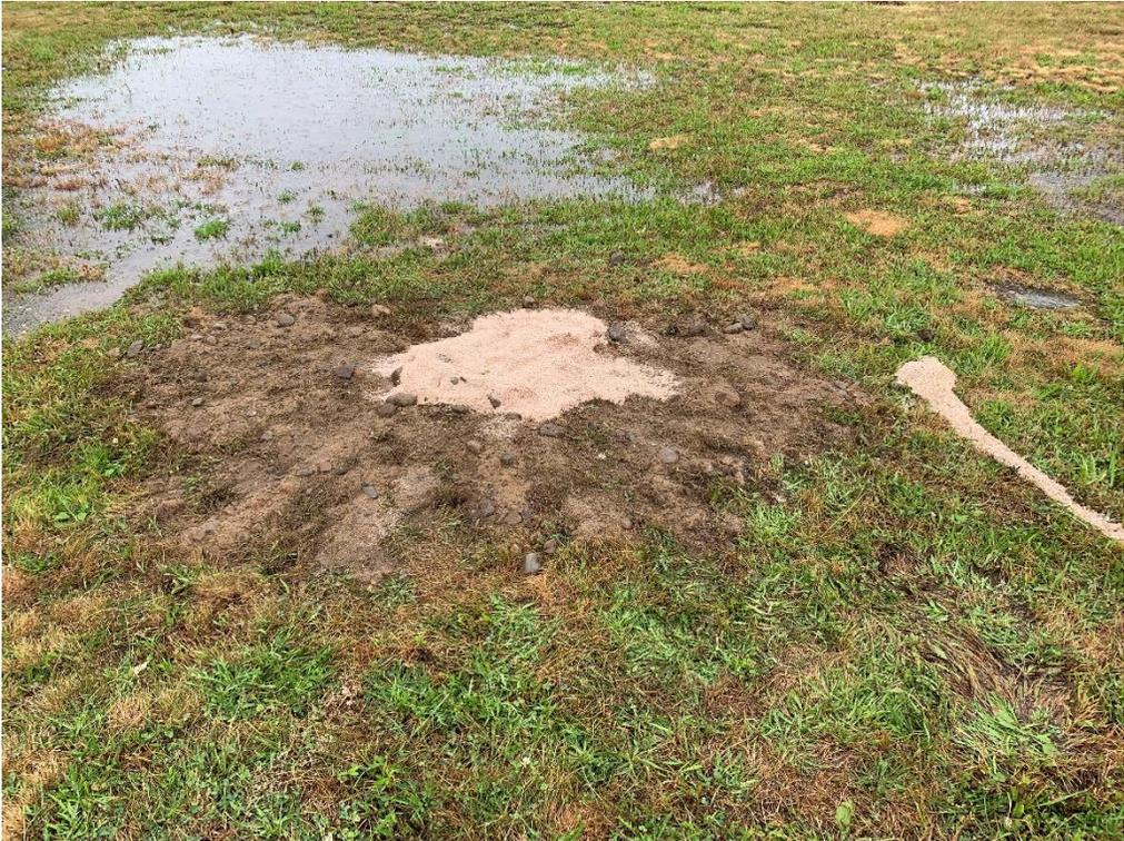
A photograph showing the site of monitoring well 15MW2 after decommissioning. The well opening is filled with a mound of light-colored sand or soil. The surrounding area is grassy with some water puddles in the background.                                |
